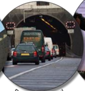
Dartford East Tunnel
